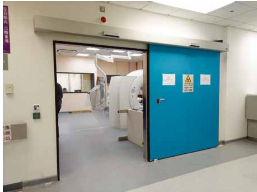
CT Scan Room No.2, A & E Department at North District Hospital
