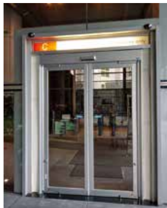
NABCO Mini Glide Door Project Lobby C, HSBC Headquarter
